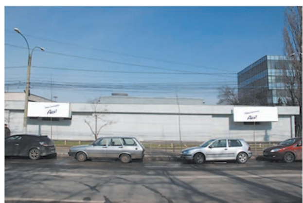
BANNER DISPLAY ON ROMEXPO HEADQUARTER FACADE
